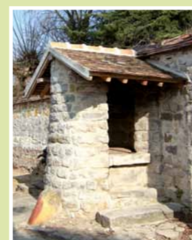
Wells rue Palizzi and rue Delort
